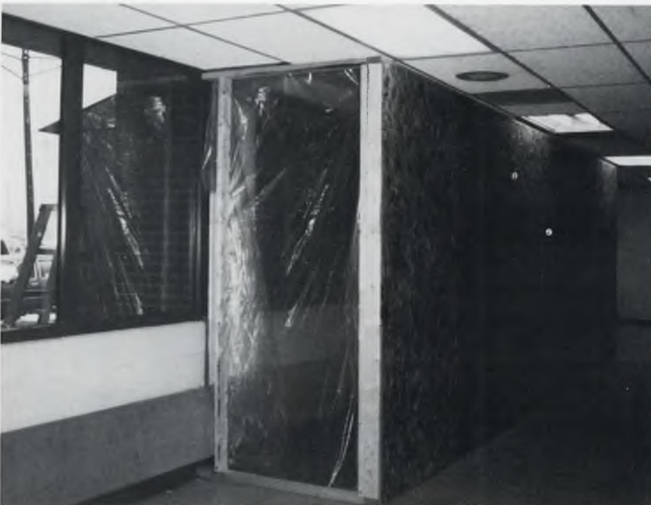
The reconstruction of the "Hole in the Wall."
