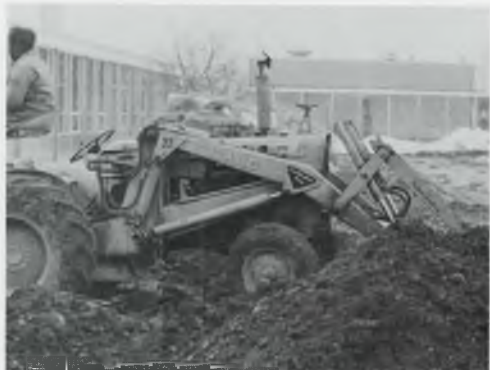
digging out material . . .
